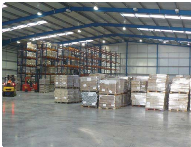
The new 30,000 sq. ft. warehouse begins to take shape
